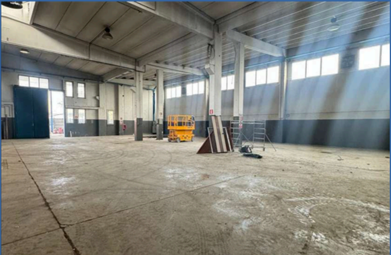
Work underway on the new Block C in 2023
